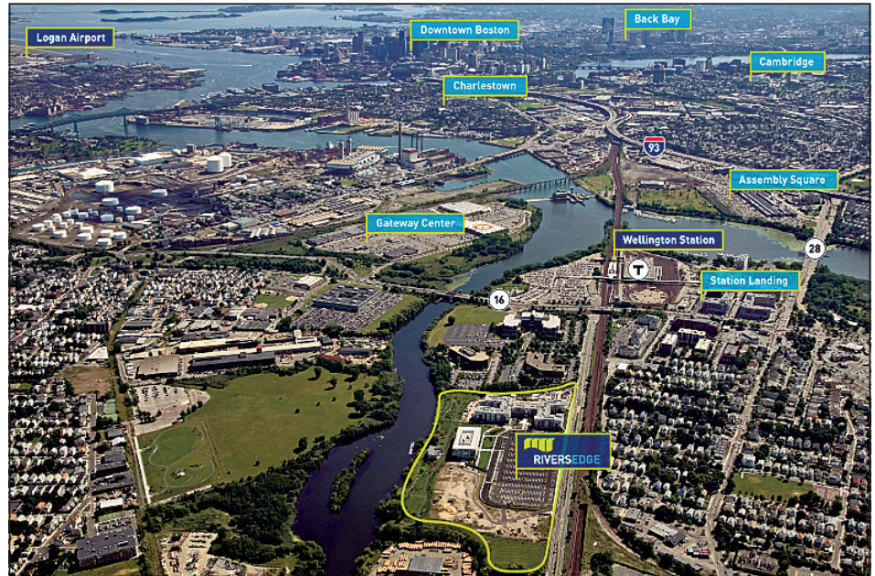
John Preotle removed thousands of tons of junk to clear the way for his new office development, outlined in green above.
